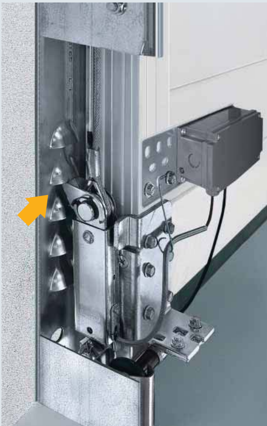
The locking hook of the arrestor kit automatically latches if the door is forced upwards.
